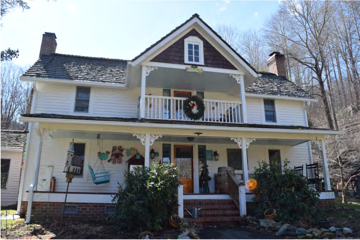
Figure 8: Facade of original house, view to the south
