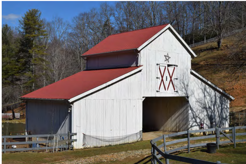
Figure 20: Barn, view to the north
