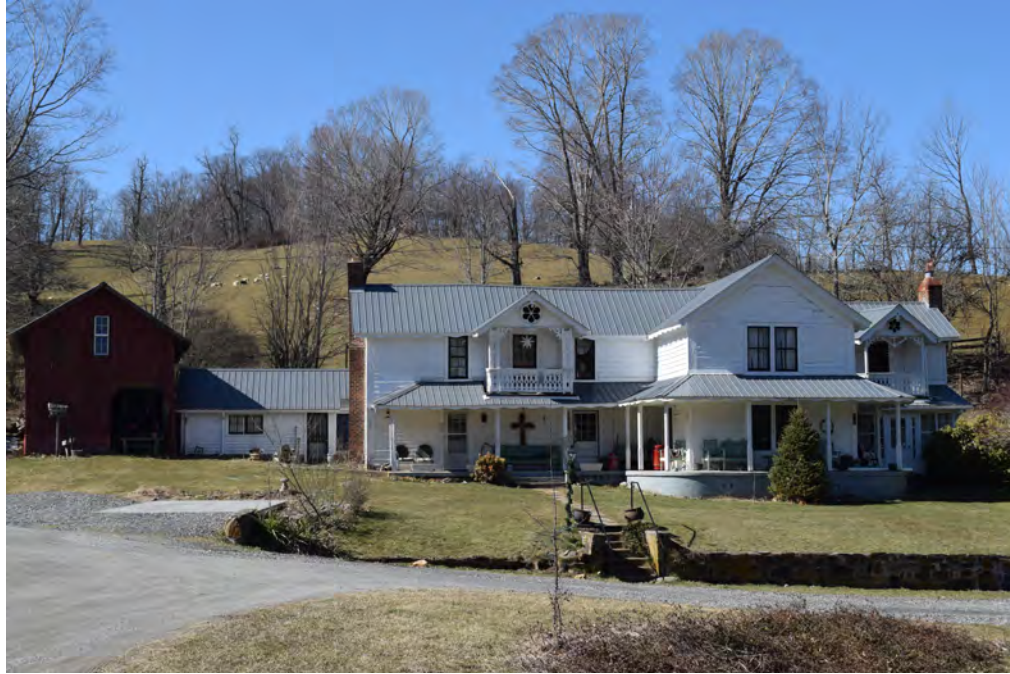
Figure 25: (WT0465): I-house at the Greene Farm, view to the north
