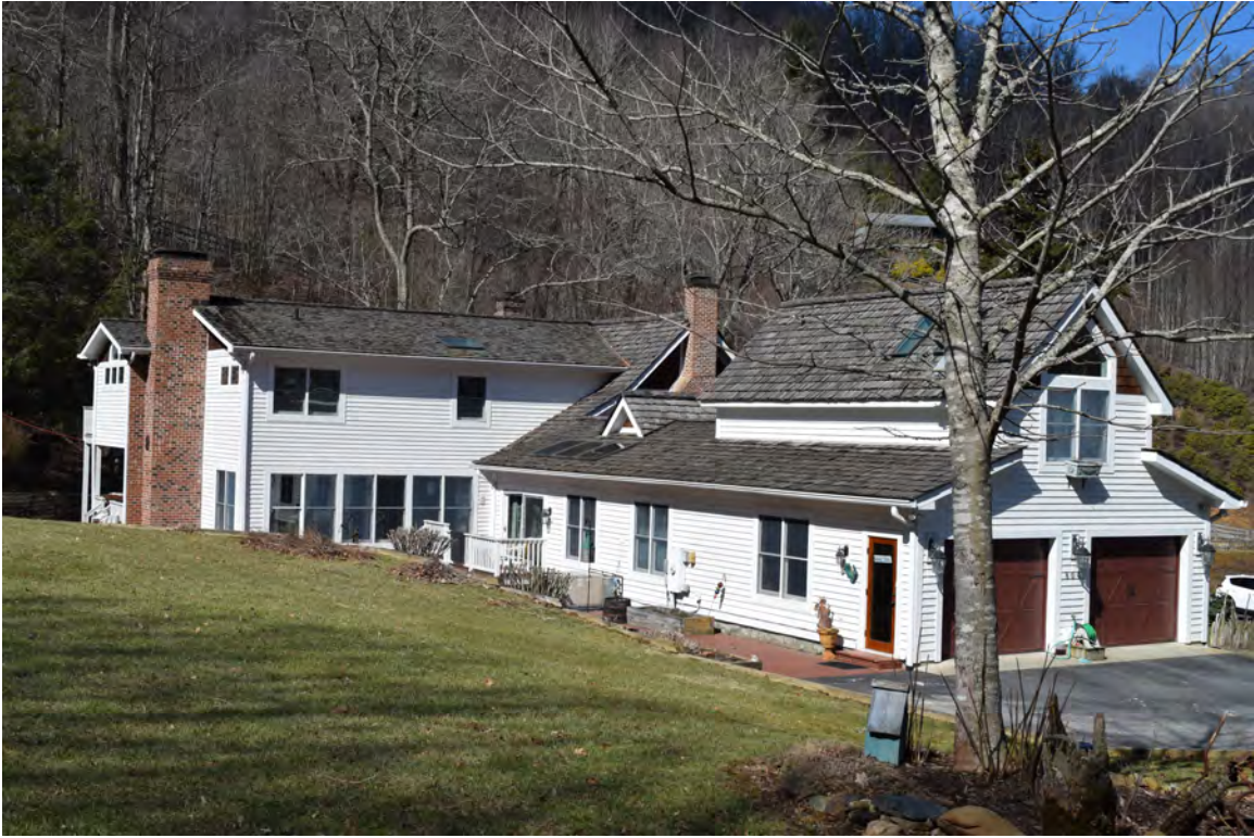
Figure 10: Rear of two additions to house, view to the northwest
