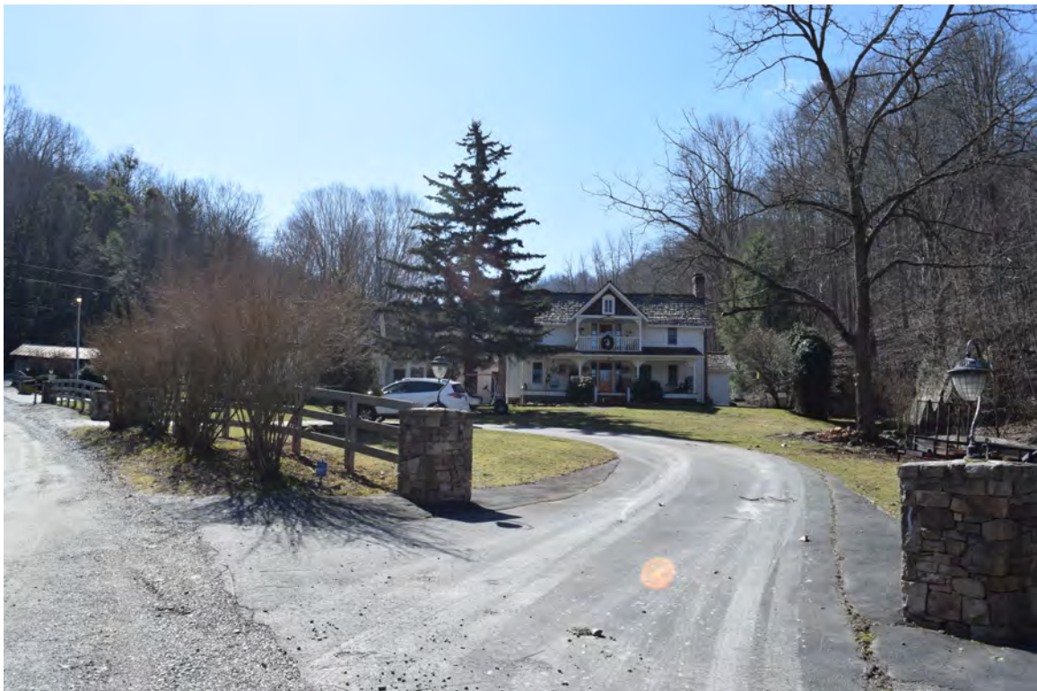
Figure 7: Approach to Samuel C. Byrd House from Justus Road, view to the south-southwest
