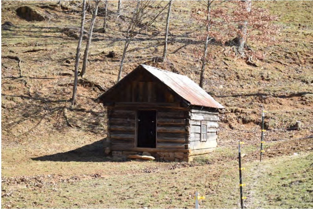
Figure 22: Log crib, view to the east
