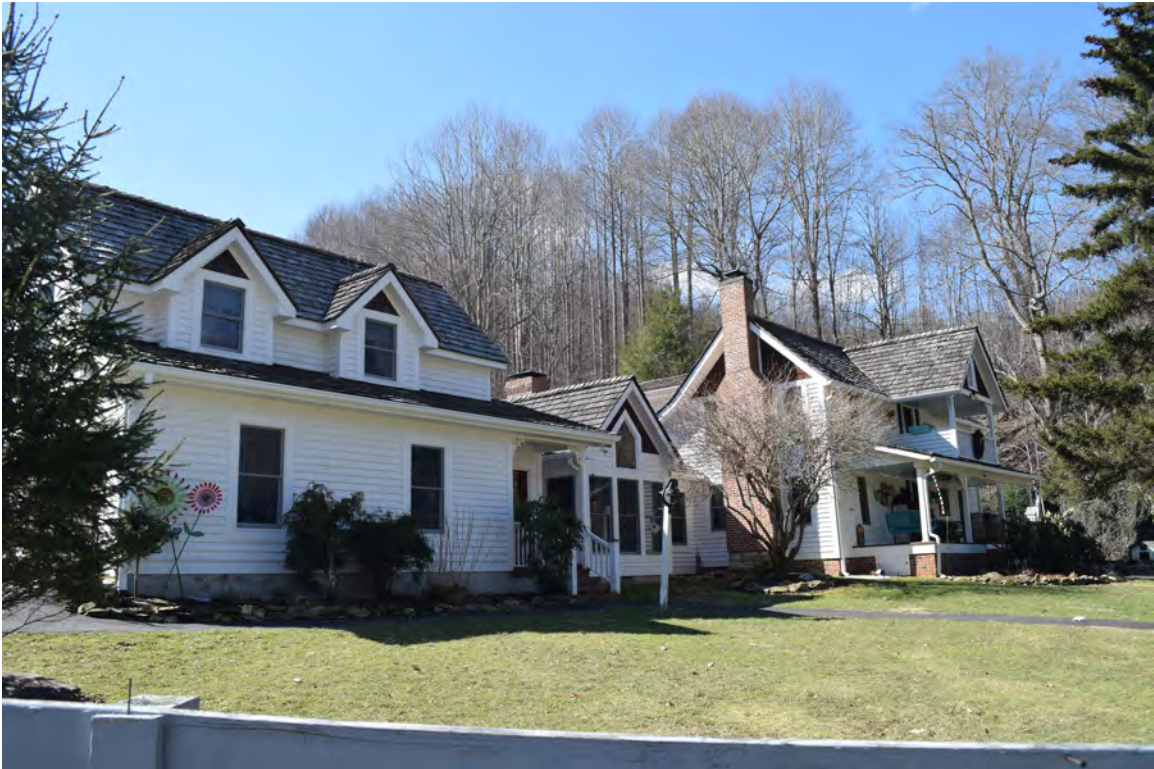
Figure 9: House with east side addition in foreground, view to the southwest
