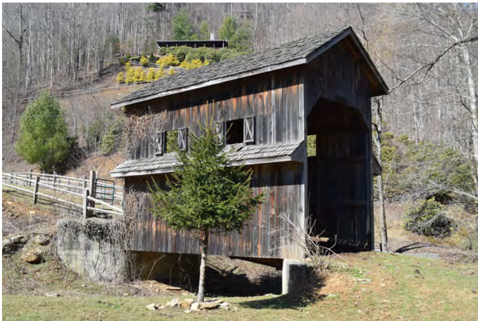
Figure 18: Covered bridge, view to the northwest
