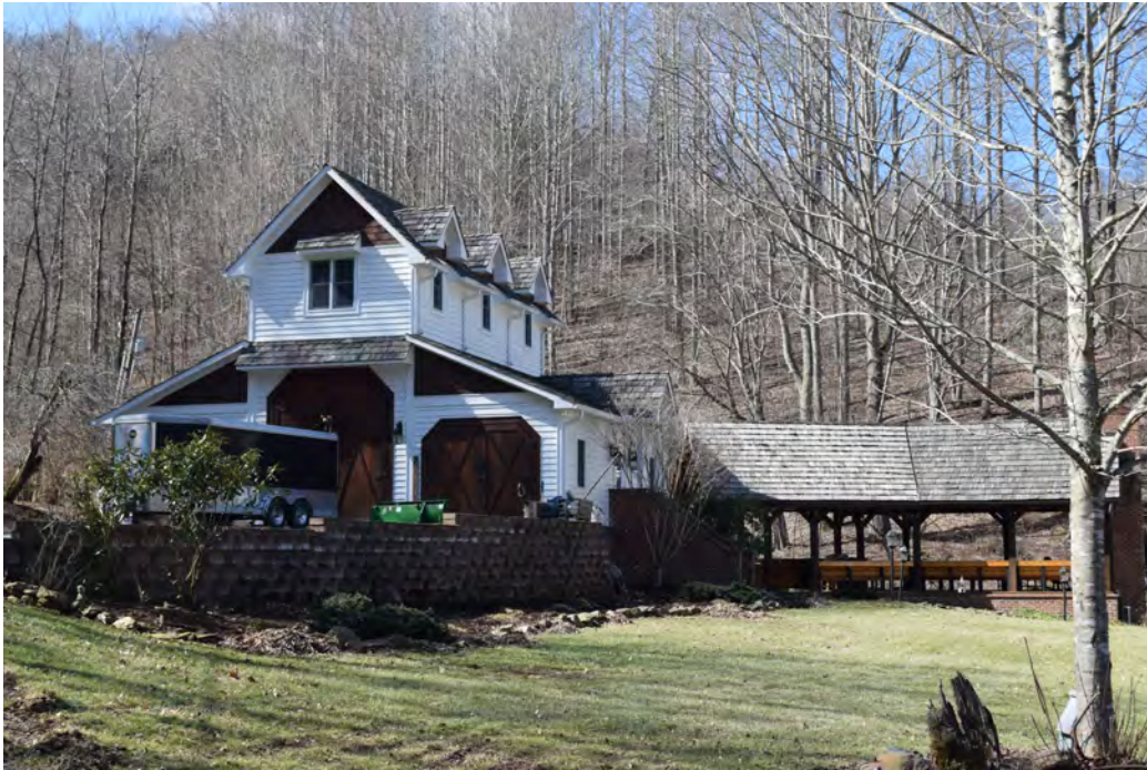
Figure 16: Garage/workshop (left) and entertainment pavilion (right), view to the southwest
